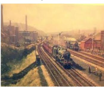
Ecclesall engine shed, to serve the Midland Main Line between London, St Pancras and Sheffield. It was used mainly to stable and service passenger and mixed-traffic locomotives for use on trains from the nearby Sheffield Midland Station. The shed was built down from Millhouses station and was easily viewed by train-spotters who would
